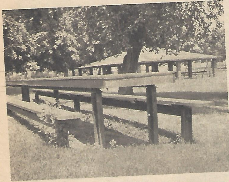
Shelbyville's Morrison Park has an abundance of tables built from interurban tracks (above). T-rails were also used as beams to support the concrete floor of the bandshell (below).
