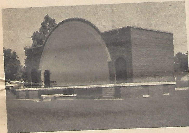
Shelbyville's Morrison Park has an abundance of tables built from interurban tracks (above). T-rails were also used as beams to support the concrete floor of the bandshell (below).
