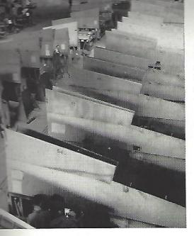
Final wing assembly department where wings are rushed to completion to keep a date with the urgent production lines.
