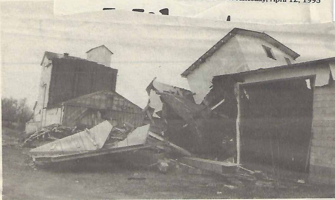
OLD MILL COMING DOWN IN MENTONE
