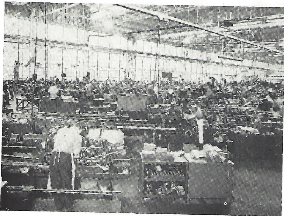
A corner of the machine shop in Bell's Buffalo plant. Latest of machine tools are employed to cut every production "corner" possible in the race to step-up output.
