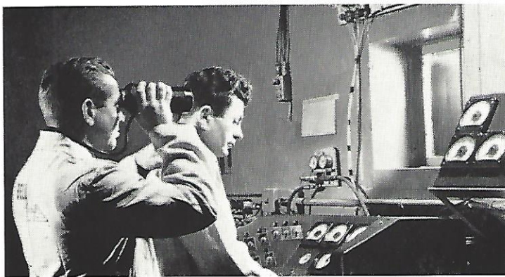
Special concrete and steel reinforced test cells permit engineers to make direct visual check of rocket engine runs.
