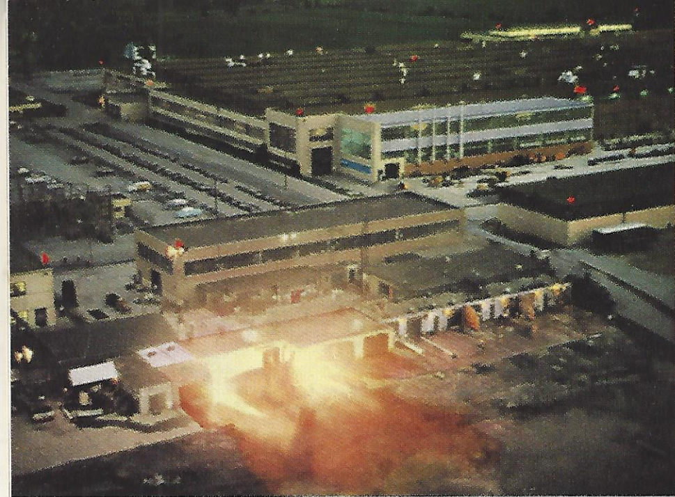
As many as 40 rocket engine runs a day are conducted in test cells at the Wheatfield Plant. Shown here is a double run, with company's main plant in background.
